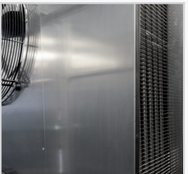
Vertical evaporator with fin spacing adapted to delay the formation of ice
